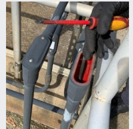
Caps on conduit at these sedimentation basins had been left open.
